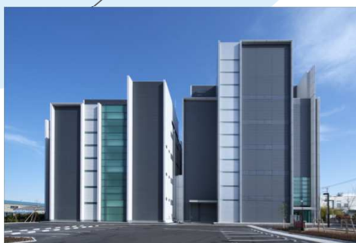
No. 2 Data Center (Yokohama)
