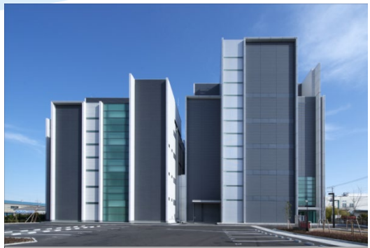
No. 2 Data Center (Yokohama)
