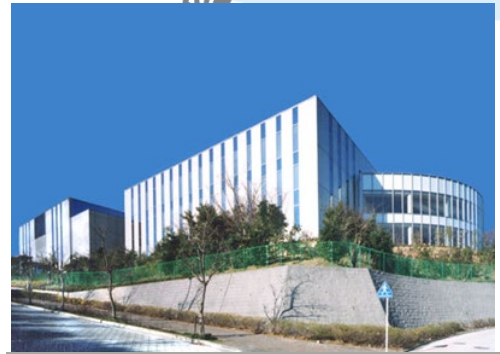
No. 1 Data Center (Yokohama)
