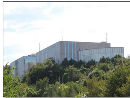
No.1 Data Center
