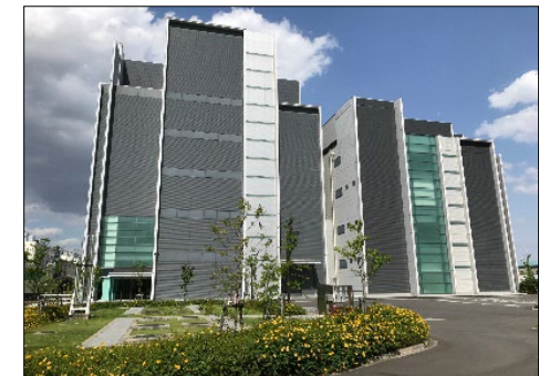
No.2 Data Center
