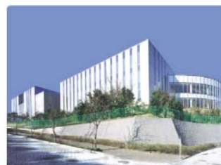
1st Data Center
