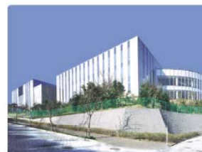
1st Data Center
