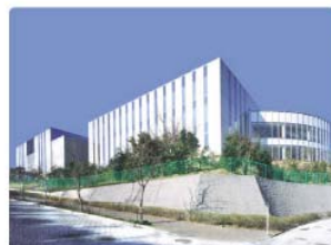
1st Data Center
