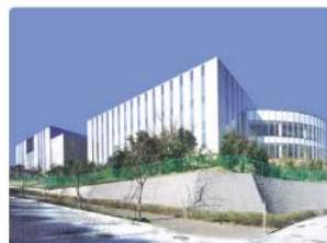
1st Data Center
