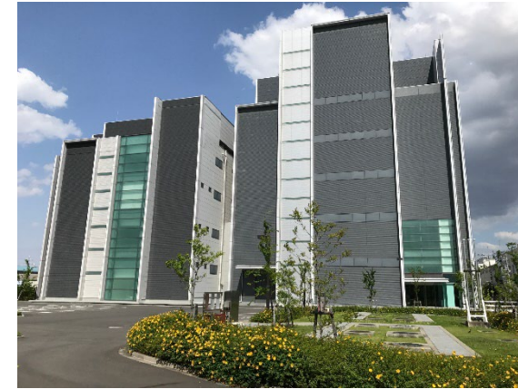
Second data center
