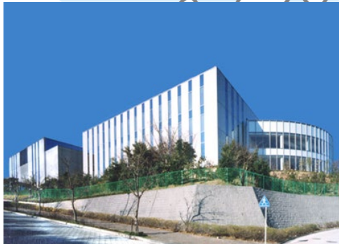
No. 1 Data Center (Yokohama)
