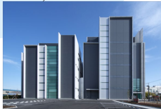
No. 2 Data Center (Yokohama)
