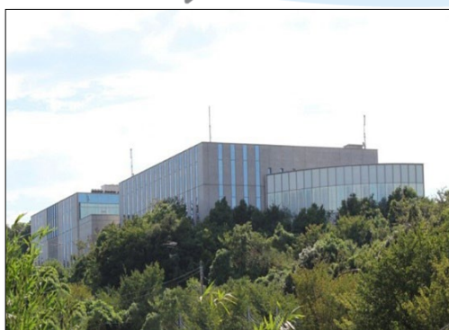
No. 1 Data Center (Yokohama)
