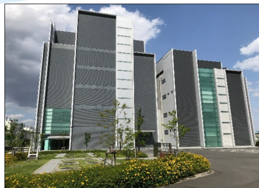
No. 2 Data Center (Yokohama)
